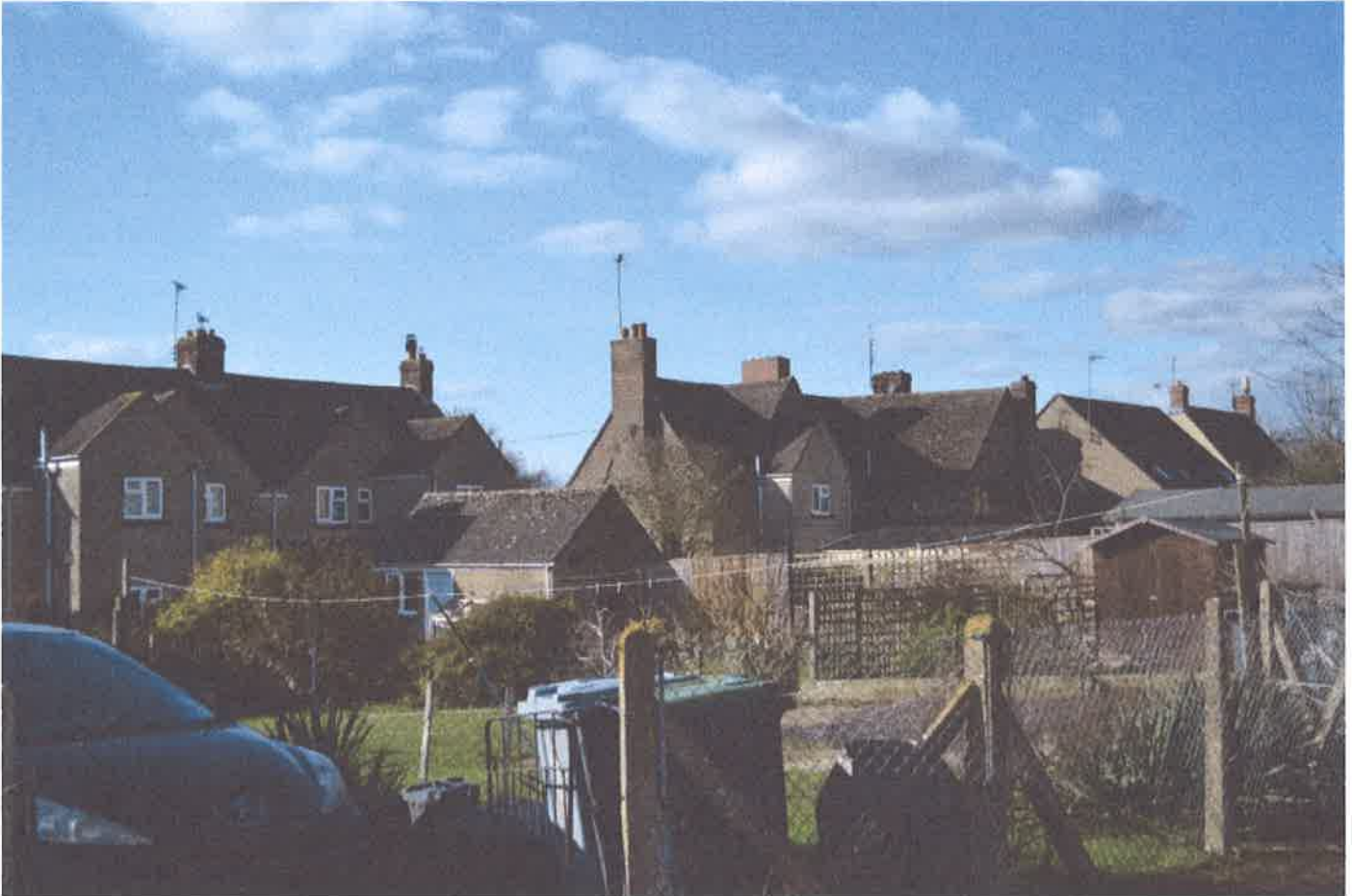
Asymmetrical elements, 'wrap-around' intersecting volumes and a mix of gables are typical of the area
